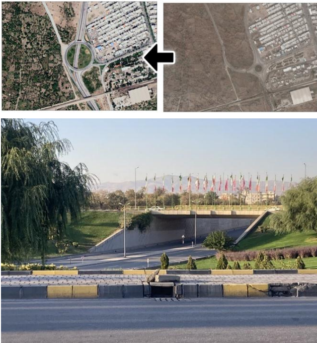
Fig. 7. Khalij-e Fars Underpass
