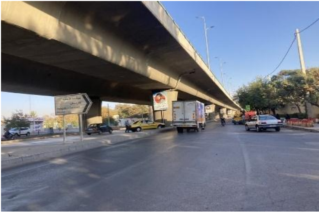
Fig. 9. Imam reza overpass
