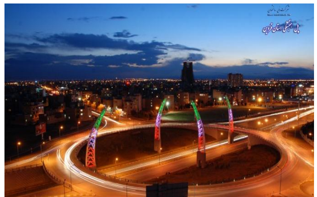
Fig. 6. Seyed hassan nasrollah underpass
