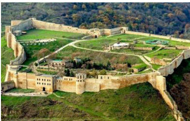
The ancient city of Darband and its surrounding fortifications and citadel, dating to the Sasanian period, were built to control the border between the northern and southern Caucasus. The strategic importance of this fortress and its walls lies in their location on the slopes of the Nabasaran Mountains in the Caucasus range, forming the only accessible passage between the sea and the mountains.
