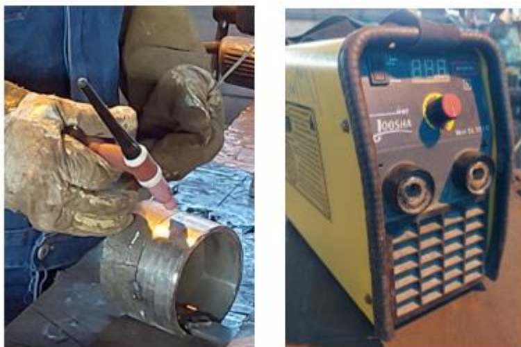
Figure 5. Pictures of welding machine and argon torch
