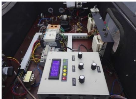
Fig. 4. The interrupter installed on the rectifier transformer.
