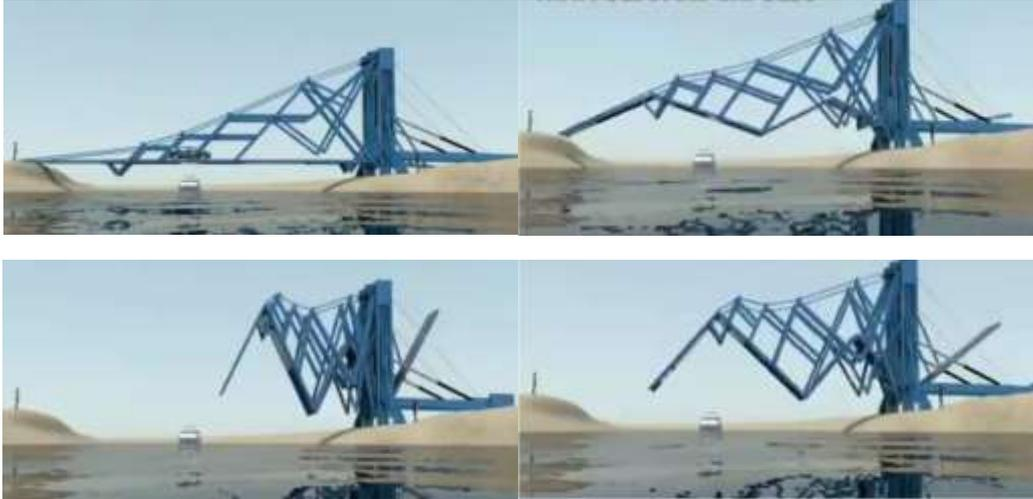
Fig.14. Operation of the Bridge
