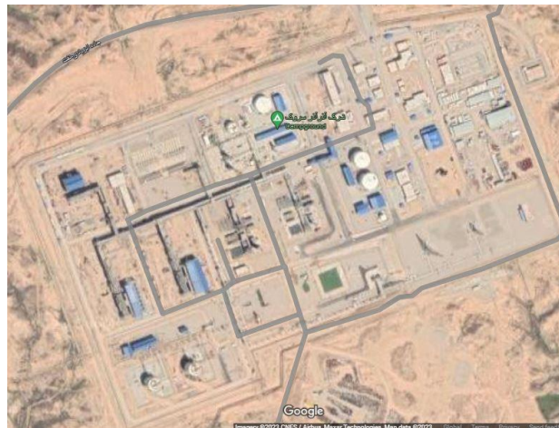
Figure 1. Sarvak Azar Central Processing Facility.
