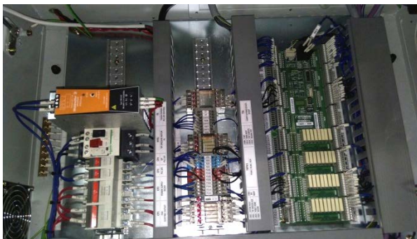
Fig.7. Embedded PLC to interlock robots with other devices
