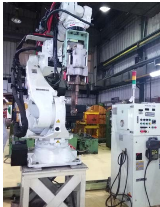
Fig.6. Robot controllers along with interlock panel
