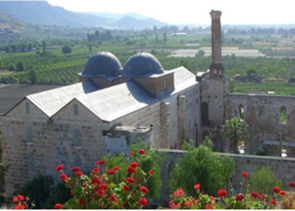
Figure.7: A view of Isa Bey Mosque in Seljuk (Goodwin, 2009:122).
