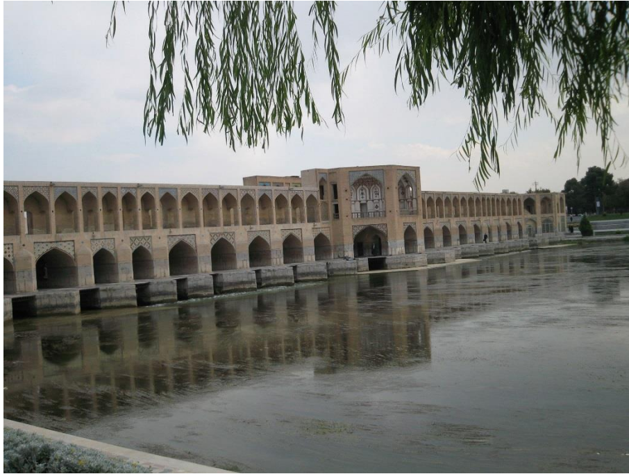
Figure (10): Khaju Bridge
