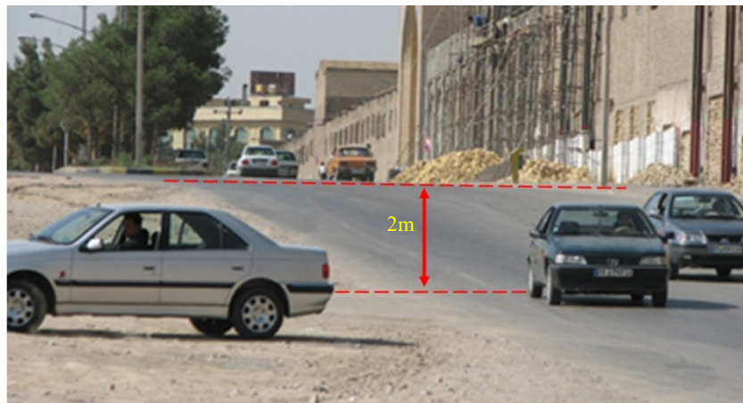
Fig 3. About 2 m subsidence in northern part of Tous Fault in khajerabie area, (Naderi and Sharifi 2018)
