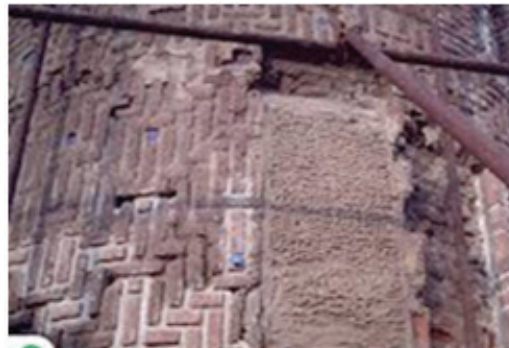
Fig. 7: Minaret of Grand Mosque in Ardabil and its layering
