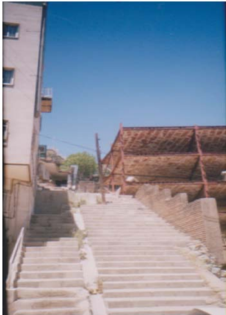
Fig. 8: reposing two heterogeneous fabrics by each other, in Ajoodanieh district, region one of Tehran municipality. (Source Authors)
