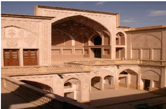
Fig. 8: The building in the second floor is set back to provide better access to the sun. Abasian House, Kashan, Iran.
