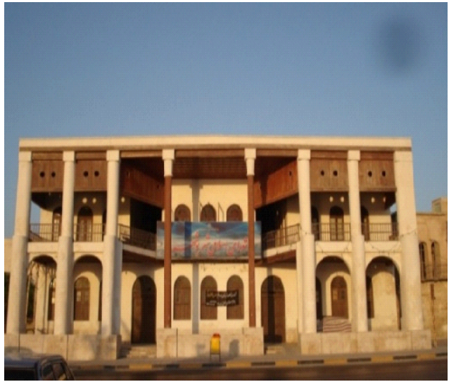
Fig.11:Large outer windows in the upper part for ventilation
