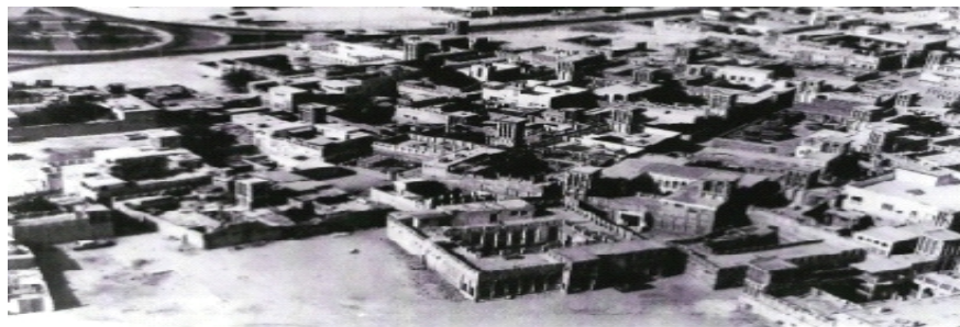
Fig.14: Dense fabric of Bastakieh neighborhood in Dubai and the wind towers built by the Iranian immigrants (source: www.bastaki.ae/image)
