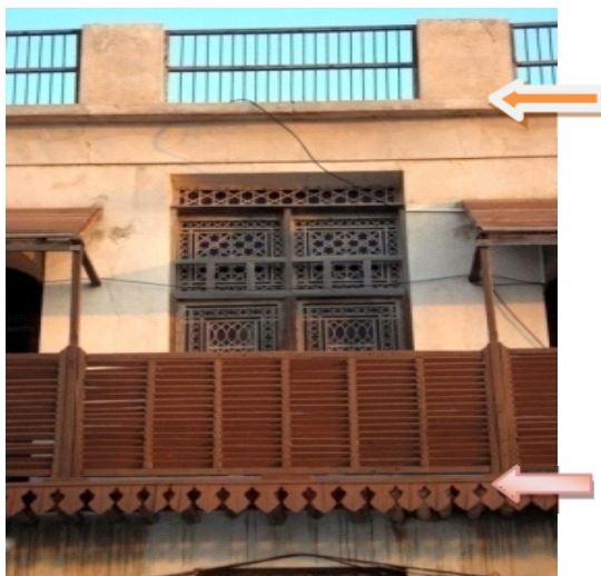
Fig.4: Some parapets in the roofs and shanashir "balconie"
