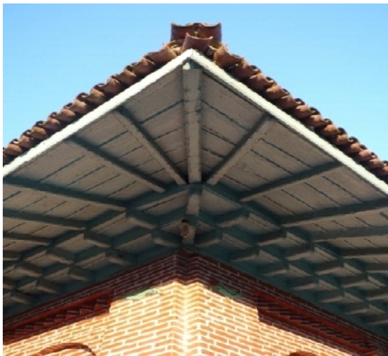
Fig.9: Wooden Beams under the Roofs
