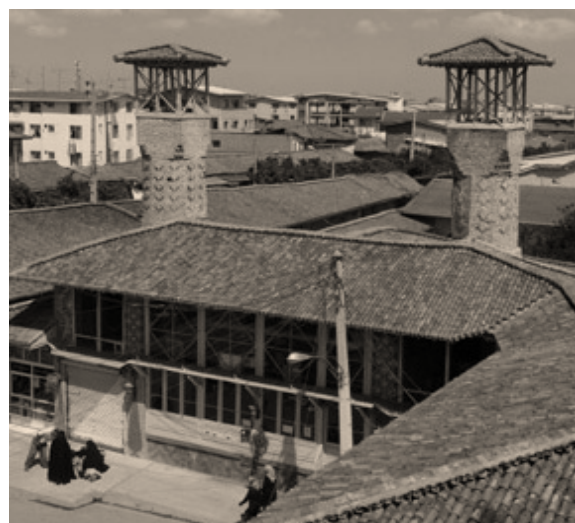
Fig.6: Gable Roofs in Panjshanbe-Bazaar Covered with Tiling
