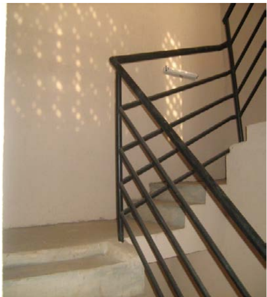
Fig.17: Stair way provided at UI hostel
