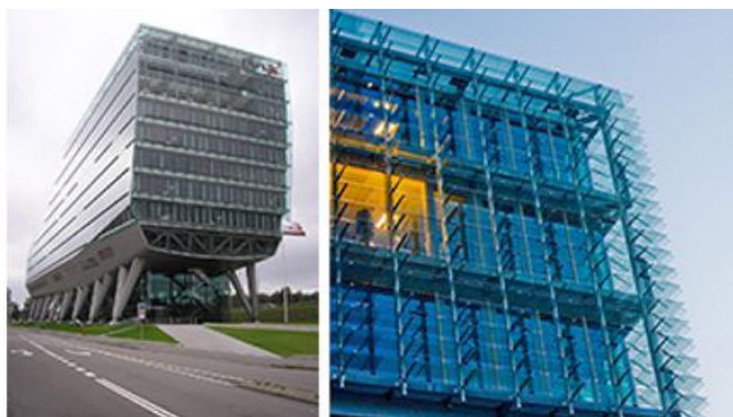
Fig. 3: Building with Double Skin Façade
