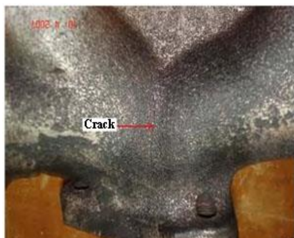
Fig. 10 Hair-line crack in thermal shock test [25].
