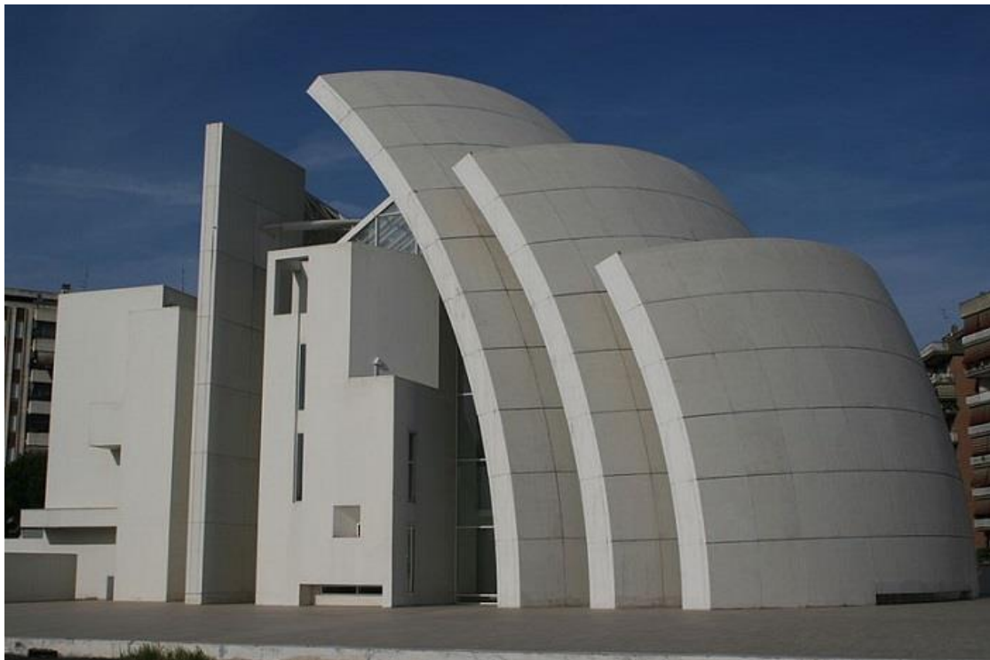
Fig. 1. Jubilee Church, Rome, Italy. In the facade of this structure, concrete is used to combine titanium dioxide nanoparticles.
