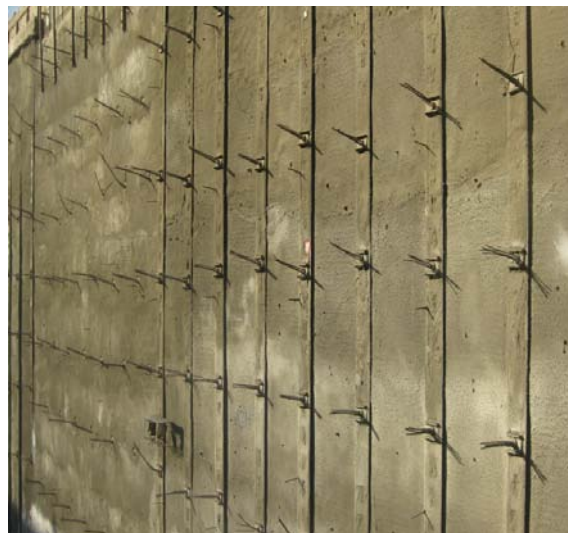
Figure 1. A view of stabilized wall by soil anchorage and steel pile
