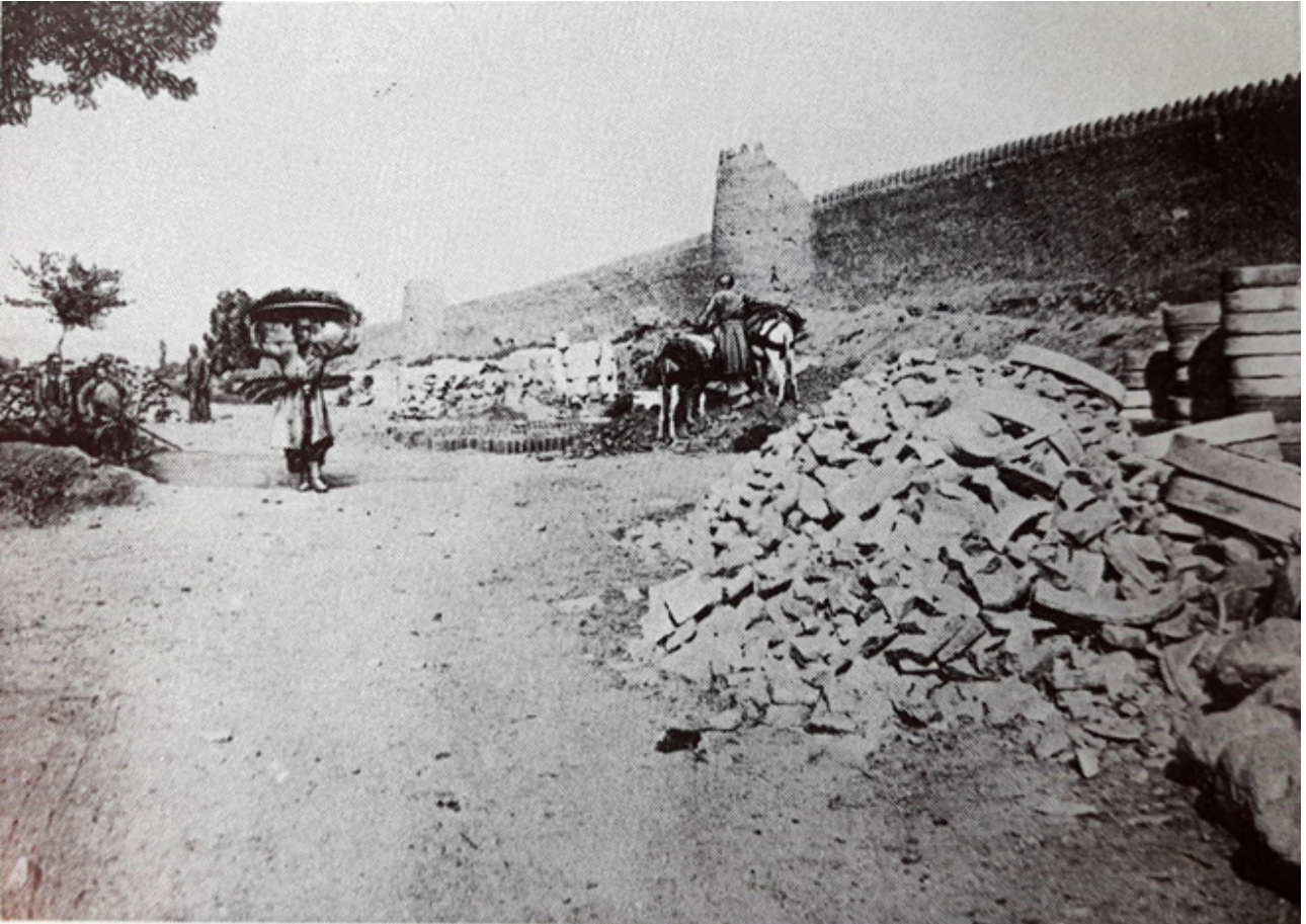
Figure 3: The tower and defensive wall of the city of Mashhad (Mahvan, 2012)
