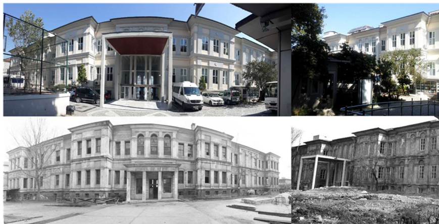
Fig. 2. Entrance of Mesfaou Findikli Campus, (photographs from before* (below) the renovation and current state (above) (*Courtesy of Mimar Sinan Fine Arts University Photography Studio) [12].
