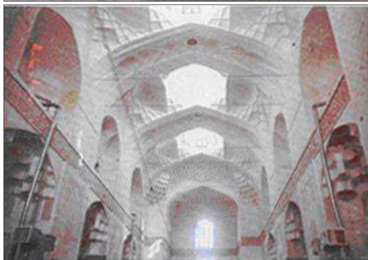
Figure 10: The mass reduction going along with hollowing the walls and the roofs at the height, (Right: The tomb of Moshtagh Ali Shah in Kerman) (Left: School of Agha Bozorg in Kashan)
