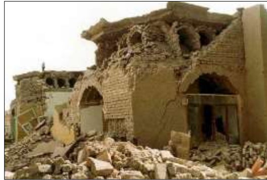
Figure 9: Bam, Konoo sazi (Build the little arch) to build a mass-reduced roof and preventing the possible movements
