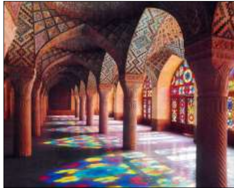
Figure 11: The reduction of mass with the use of heavy columns, the elimination of voluminous or bulky walls and the use of light shells or covers in order to “khancheh poosh” the roof. Shiraz
