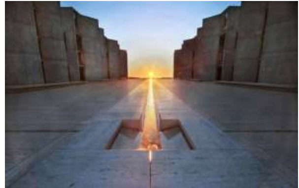
Figure 1. Louis I. Kahn, Salk Institute for Biological Studies, La Jolla, California, 1959-65 (Source: Pallasmaa, 2009: 101)
