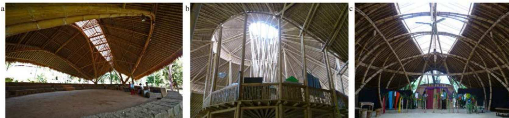
Fig. 9. Green School structure system; (a) Arches in the main hall “Mepantigan”; (b) Surface structure in main building “The heart of Green School”; (c) Bamboo arches in the class room [27].
