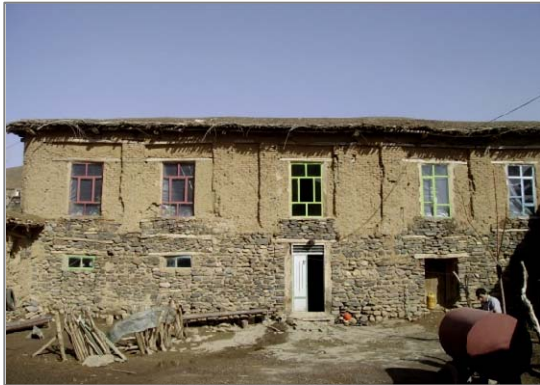
Figure (5): the lord house in 'soynas' made of a combination of adobe and stone
