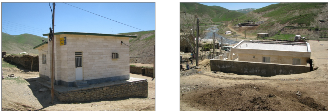
Figure (15): communication center and clinic building in the village
