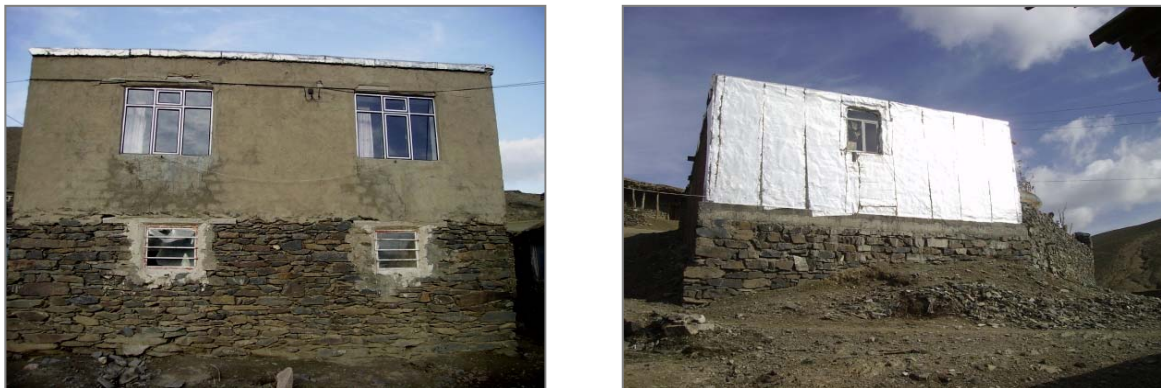
Figure (13): applying cement plaster and bitumen moisture insulation on the walls
