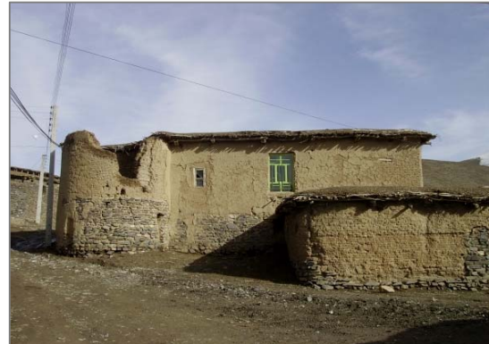
Figure (5): the lord house in 'soynas' made of a combination of adobe and stone
