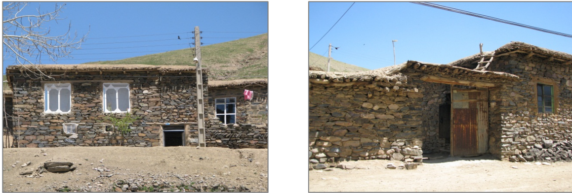
Figure (14): various shapes of metal door and window frames which are incompatible with the visual historical context
