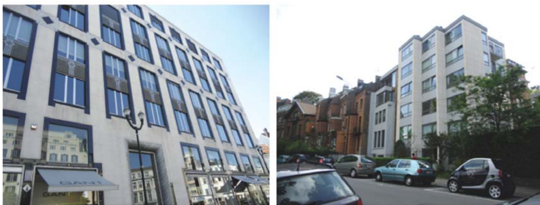
Fig. 30: Anomaly of modern architecture in Brussels 1999; any different from Tehran!
