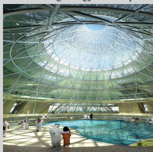
Fig. 19 . Natural lighting Staggered cones bring daylight in addition to side facades.
