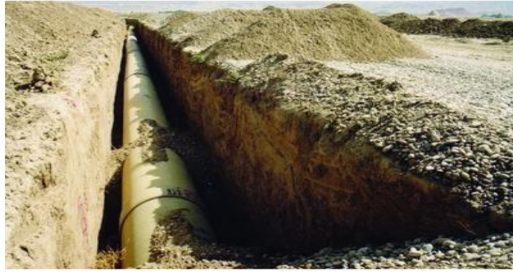
Fig 9. Execution of the GRP pipeline
