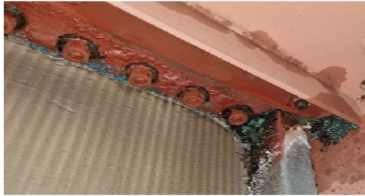
Figure 7: Corrosion of parts of the cooling cooler
