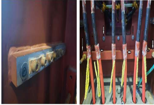
Figure 2: Corrosion in the electric motor power panels.
