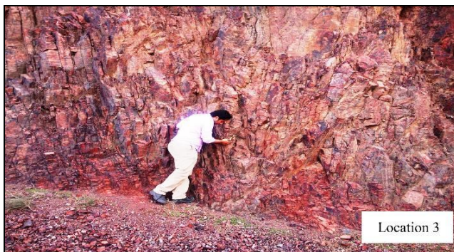
Figure 10. A view of the joint survey in Station 3
