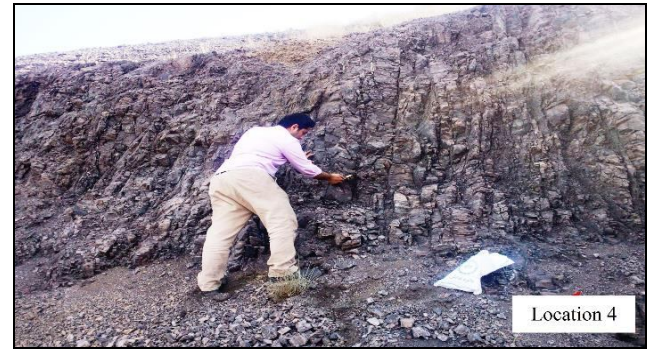
Figure 12. A view of the joint survey in Station 4
