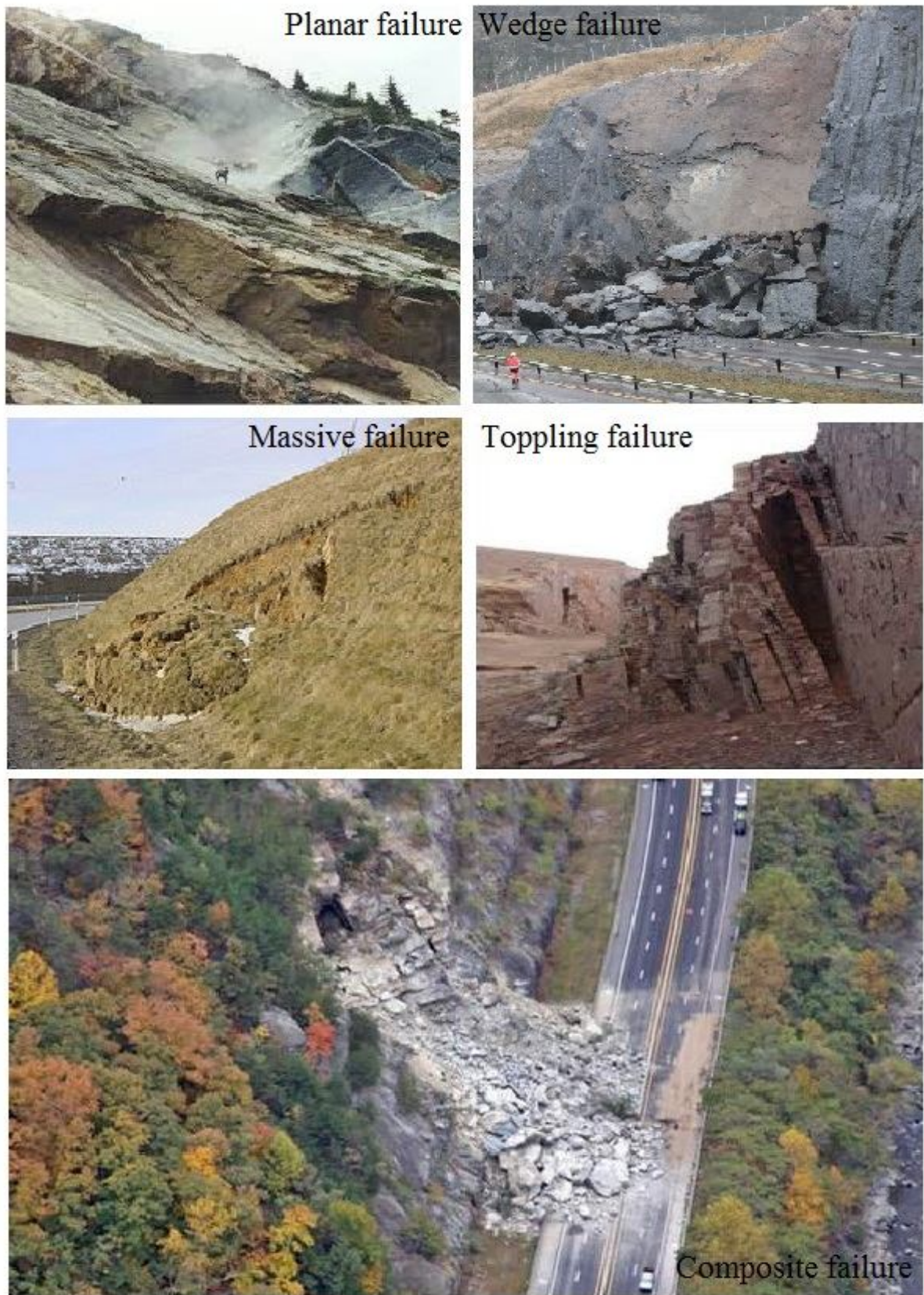
Figure 5. The topic examples for different type of the failures occurred in rock slopes (Source: Internet/Google-image)
