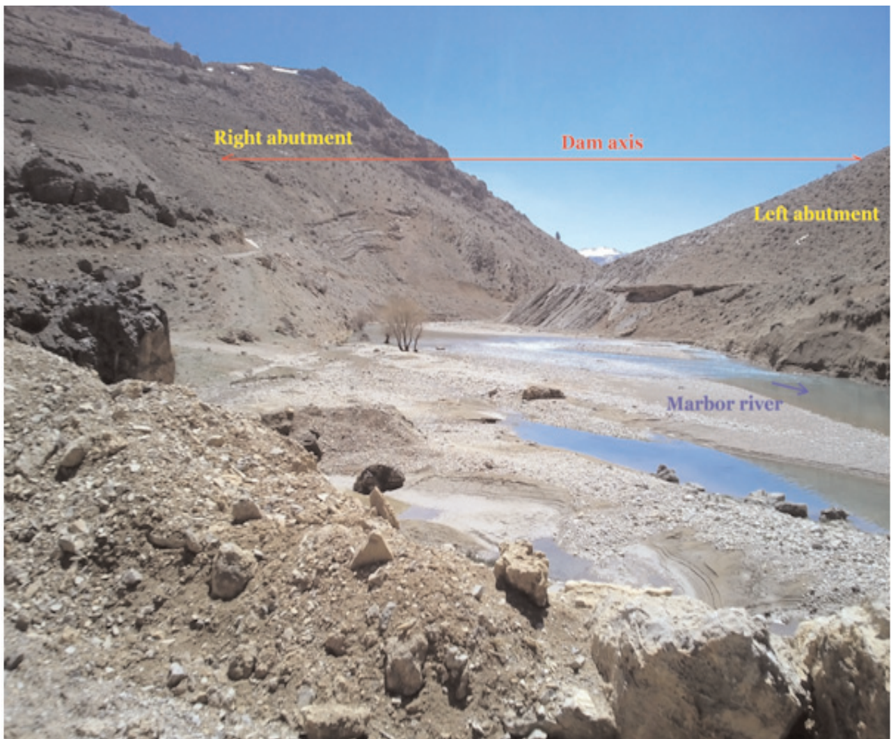
Figure 4. Dam axis (View to the south)
