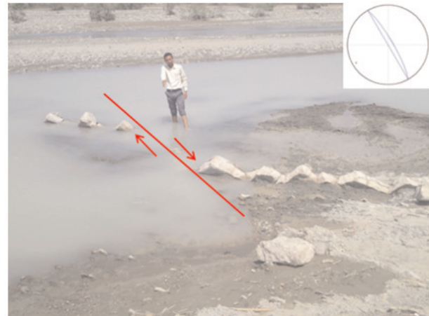
Figure 13. fault with right-hand separation at axis dam, a separation of about 2 m (see to the North East)
