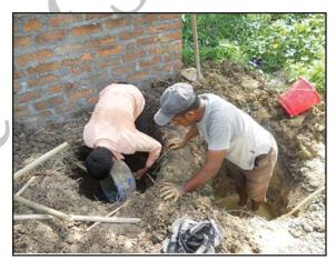
Figure a. Fitting a water pipe in B2
