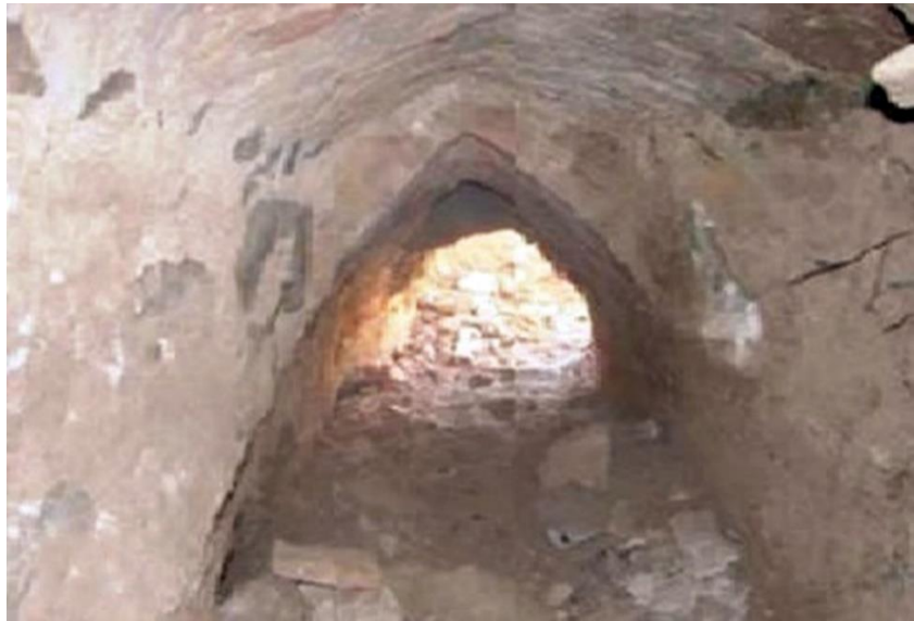
Figure 5: Secret corridor in the western slope of Tos-i Nowzar Castle (Author, 2022).
