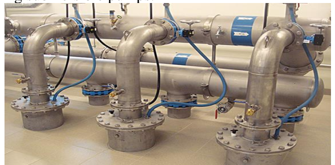
Figure 3. Vertical pumping station using floating pumps.
