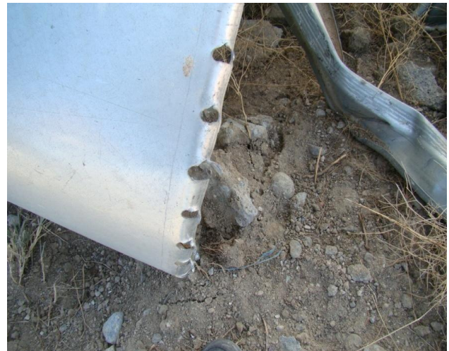
Figure 2. Rupture of shell in junction of strikes
