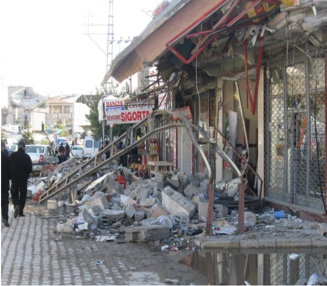
Figure 15. Collapse of an electrical pole due to collapse of adjacent building
