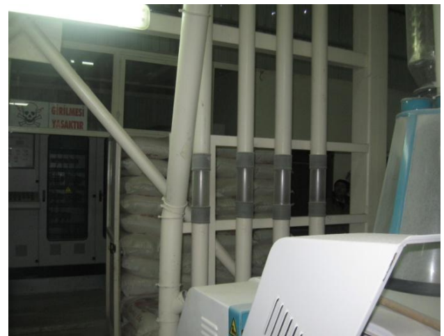
Figure 10. Undamaged pipes with flexible joints
