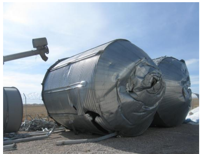
Figure 3. Collapsed silo type "B".
