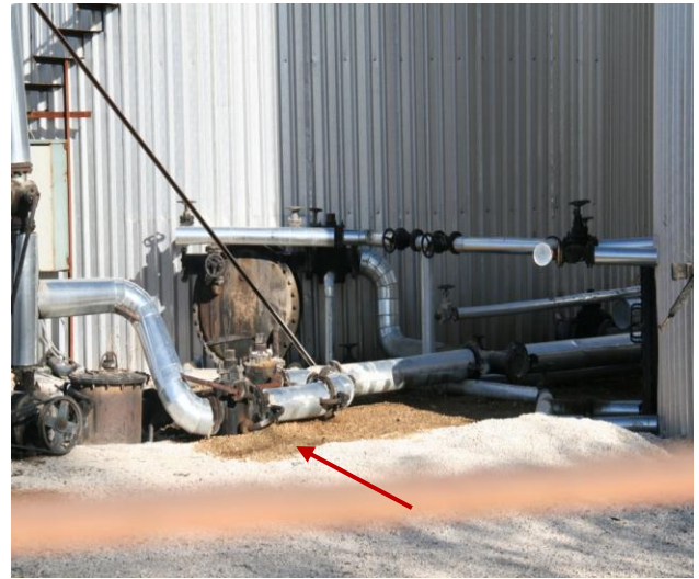
Figure 7. Repaired connection of piping system of cylindrical tanks
