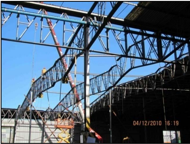
Fig. 20. Damaged warehouse being fixed
