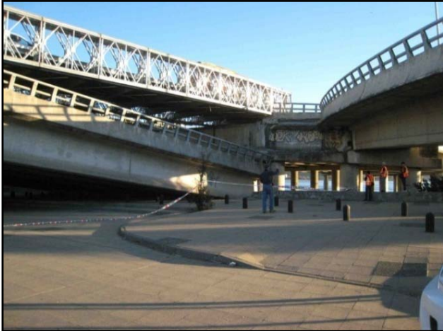
Fig 8. Juan Pablo Bridge - bailey bridge installed as a temporary fix
