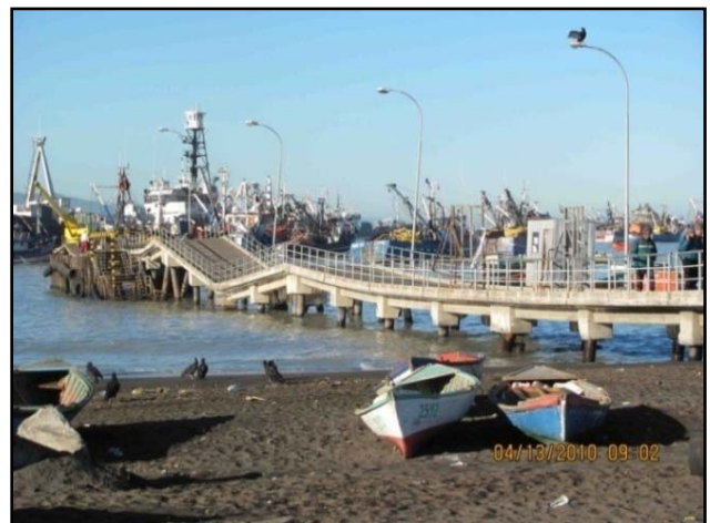
Fig. 19. Fishman pier damaged
