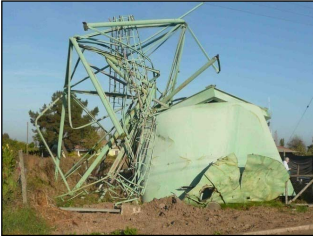
Fig. 25. Collapsed water tank (Eidinger)
