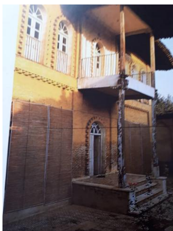
Fig. 8.Taghavi house, mat roller shades in southern windows, Ghajar period (Source: New life - old structure a selection of valuable structures, 1372).
