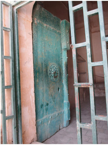
The main entrance door of the building of Imamzadeh Ghasem and Zaid Azna, Lorestan, Iran (Photo by Authors).
