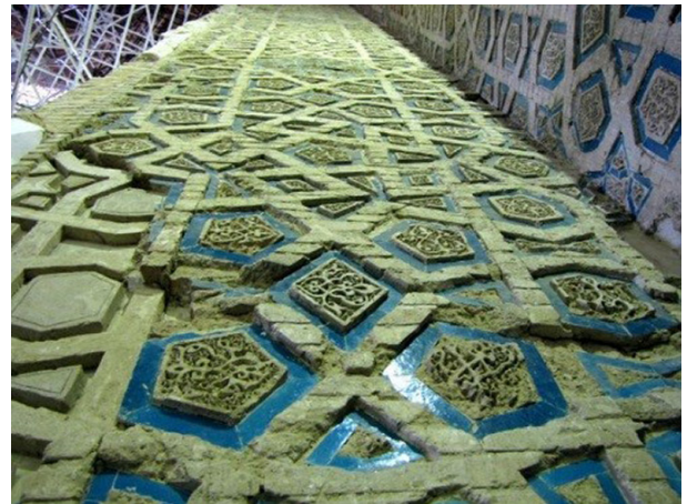
The Combination of colored pottery tiles and pottery and glazed tiles, decorations under the dome of Soltanieh, Soltanieh, Zanjan, Iran, Ilkhanid period
