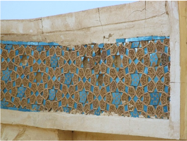
The Combination tiles with Naghshin pottery, under the arch of the entrance of Imamzadeh Qasim and Zeyd Azna, Lorestan, Iran
