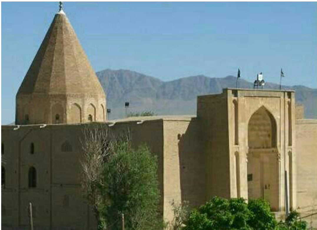
Fig. 1: 16 cracked Ridge domes, building of Imamzadeh Qasim and Zeyd in Azna, Lorestan, Iran, Photo by Mr. Farhadi's Archive of Imamzadeh Qasim Azna village, Iran.
