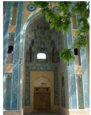
Elevated entrance lintel with Outstanding Muqarnas, Entrance lintel of Natanz Grand Mosque, Isfahan, Iran, 704 A.H.
