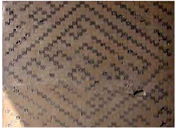
Simulation of a brick design on the plaster of Pir Bakran tomb, Falavarjan, Isfahan, Iran, Ilkhanid period
