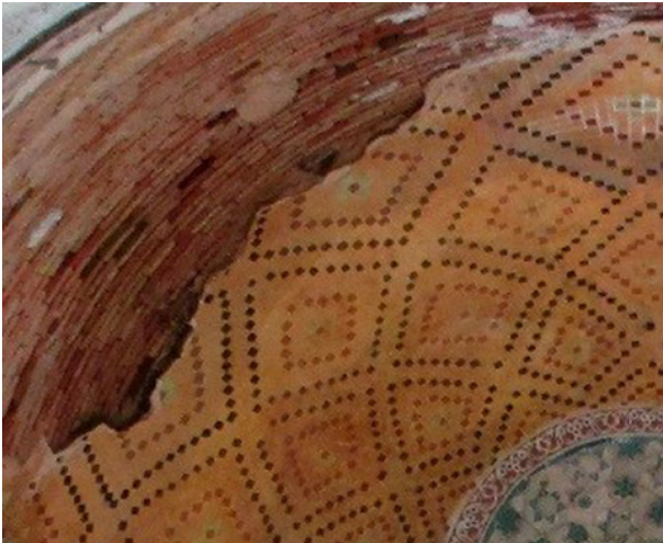
Brick design on plaster, under the dome of Imamzadeh Qasim and Zeyd in Azna, Lorestan, Iran
