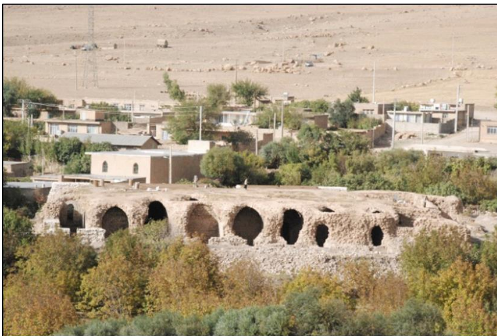
Figure 1: General view of Zij Manijeh building
