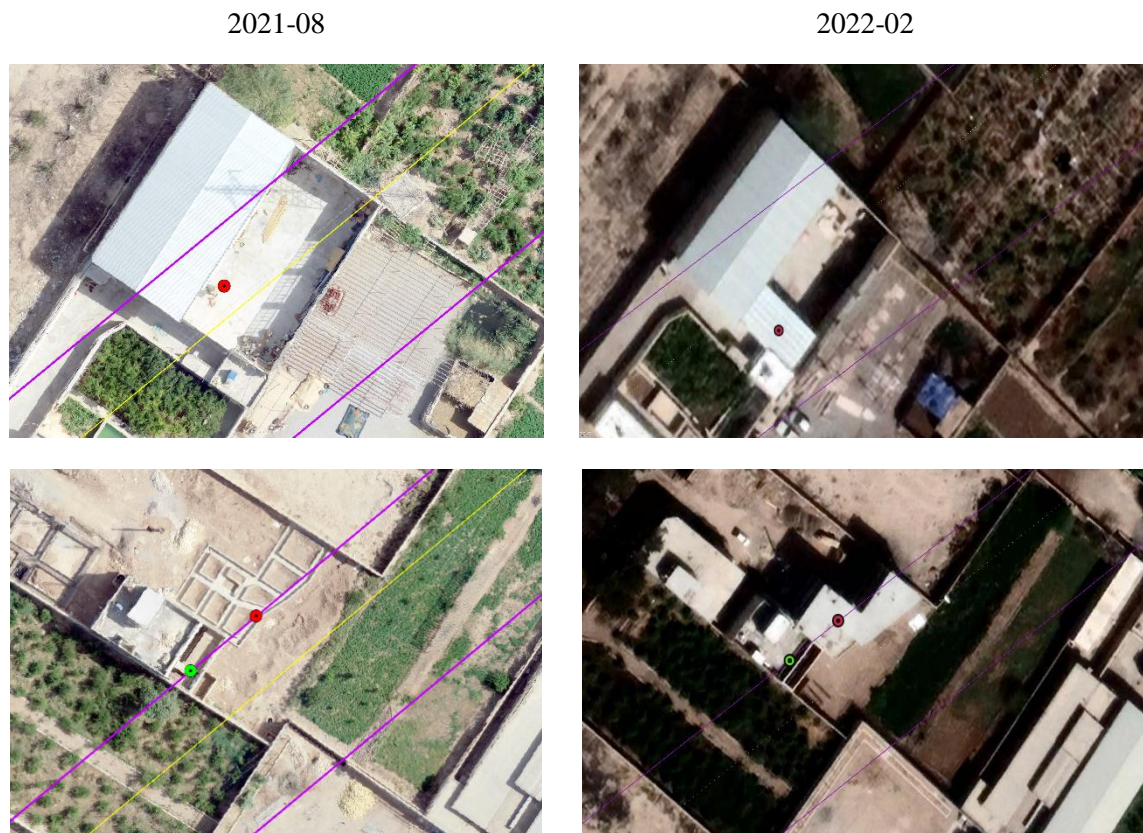
Figure 15. Construction changes during a year
