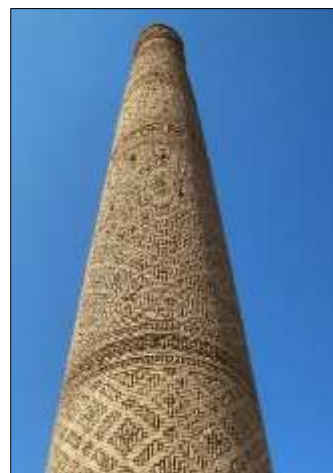
Figure 5: Khosrogerd pylon in Sabzevar
