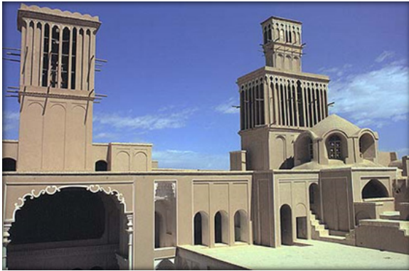
Fig.1: Windcatcher in vernacular Iranian architecture
