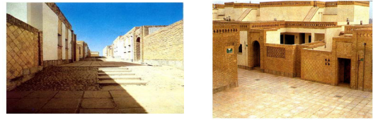
Fig. 2: Houses designed in accordance with the climate and culture of each place (source: Armanshahr counselor Engineers, 2009, 46)
