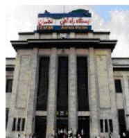
Fig. 6: Railway station Tehran
