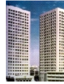
Fig. 11: Saman residential tower
