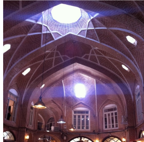
Fig. 3: Historic Bazaar of Tabriz with an emphasis on the roof function.
