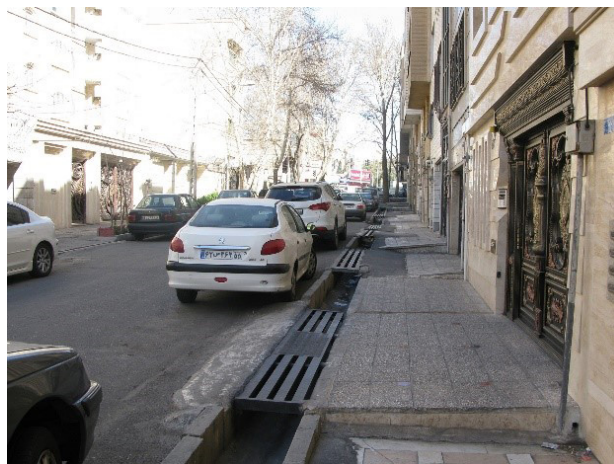
Fig. 1: The presence of frequent one-steps enhanced trip hazards.
