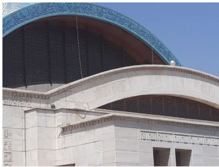
Fig.3: A close-up of translucent panels in the exterior facade
